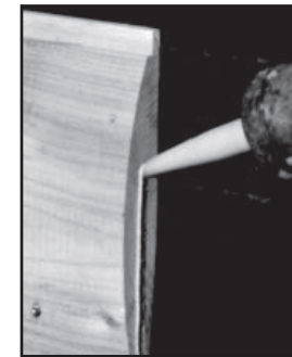
"Beading the joint" #A
